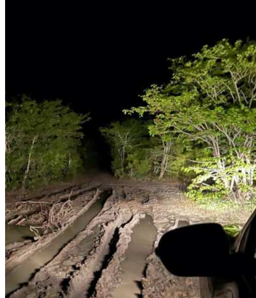
The roads in Mabalane District are often in poor condition - like this road the MSLI team was on to reach Anexa Jojo school.
