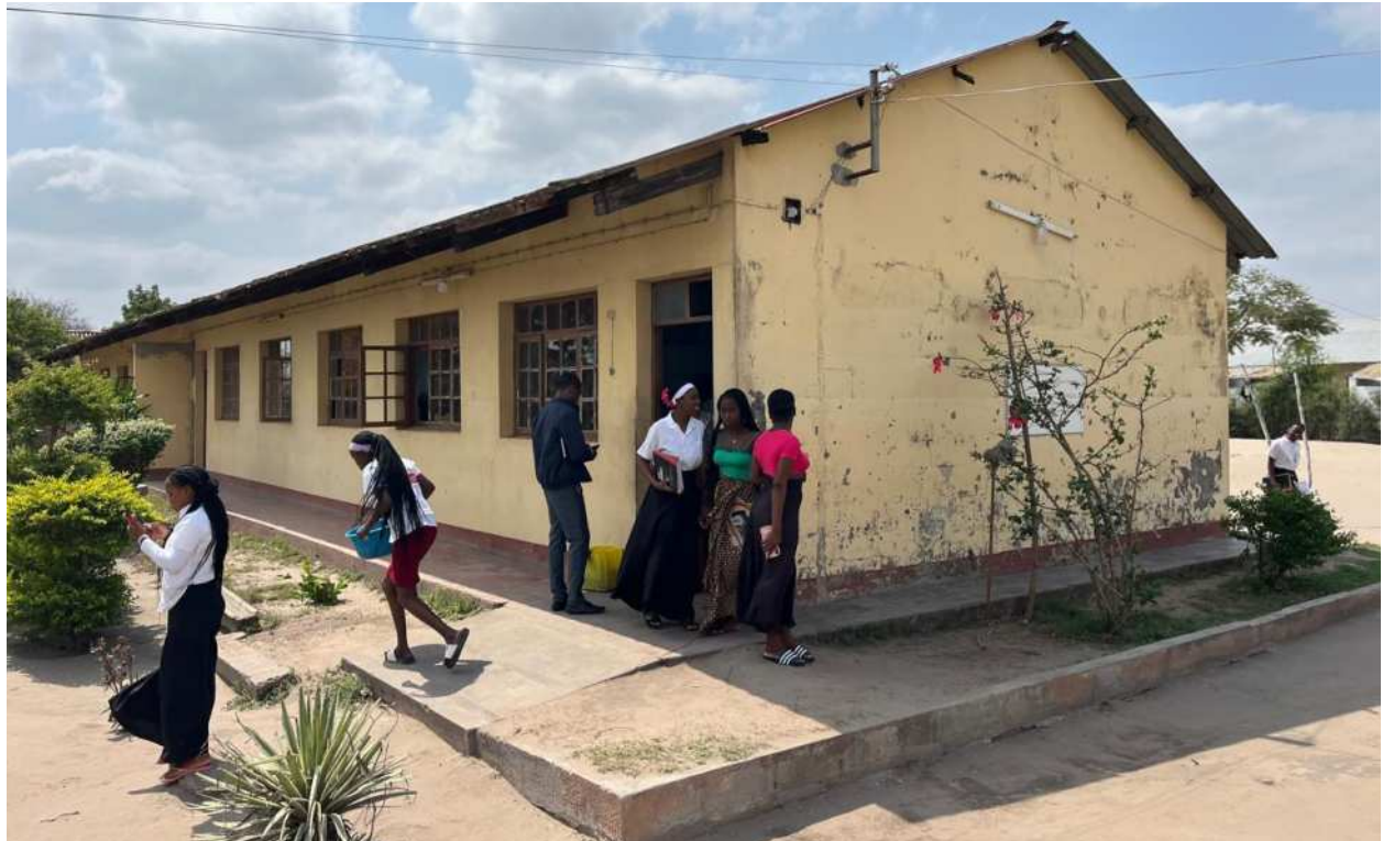
The Hókwè boarding house is located right next to one of the larger secondary schools in the area (Hókwè Secondary School), enabling students from far away villages to attend.
